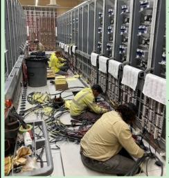
Significant progress was made in the AC Relay House to complete the interface wiring for alarm, control, and protection circuits and relays.
